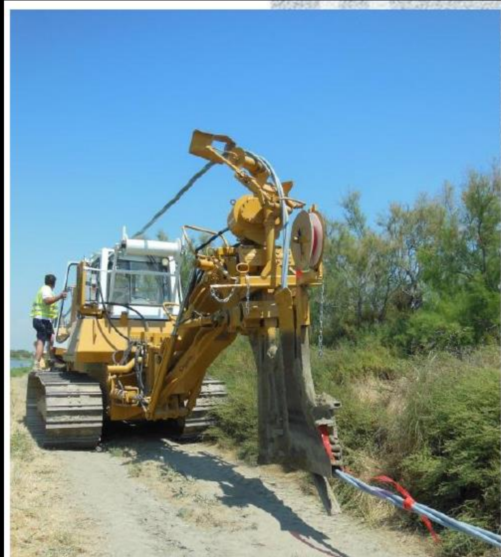
Machine used to bury electric cables
