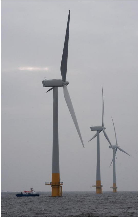
Figure 34 – Offshore wind turbine Image credit MCS/Malcom Watson
