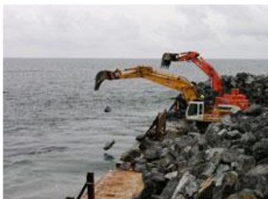
Placement of boulders
