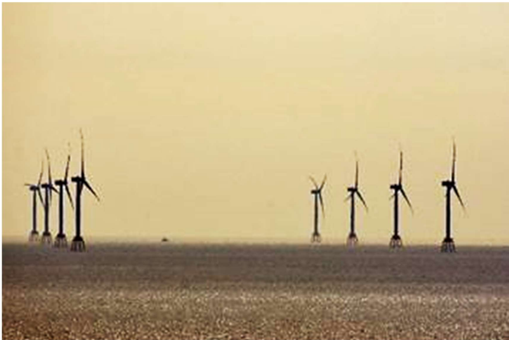
Wind turbines on jacket-type foundations. Beatrice offshore wind farm in north-east Scotland (photo : B. Guichard / Office français de la biodiversité)
